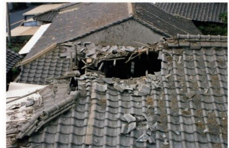
Hole in a tiled roof caused by a ballistic projectile from a volcanic eruption
